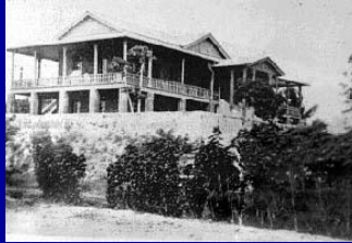
Yap – Japanese governor's house atop Spanish fort
